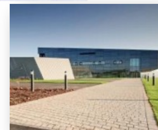
Dalton Cumbrian Facility
